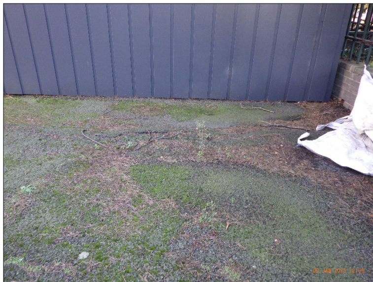
Figure 4 - Damage to car park
